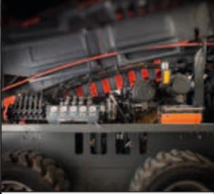
Simplified routing of cabling and hosing
