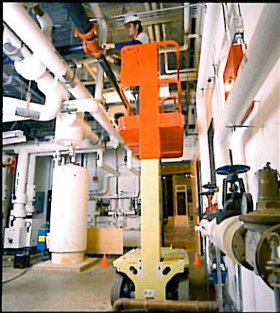
The 1.26 m x 0.69 m (Interior) platform can hold up to 230 kg.
